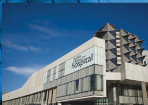
Fiona Stanley Hospital
